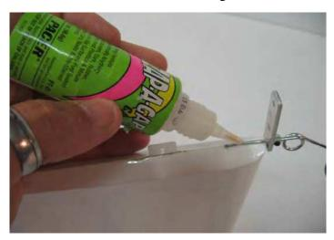
$\square$  step 5 Insert the three hinges in their appropriate slots of the rudder, and glue them with some drops of thin CA.
